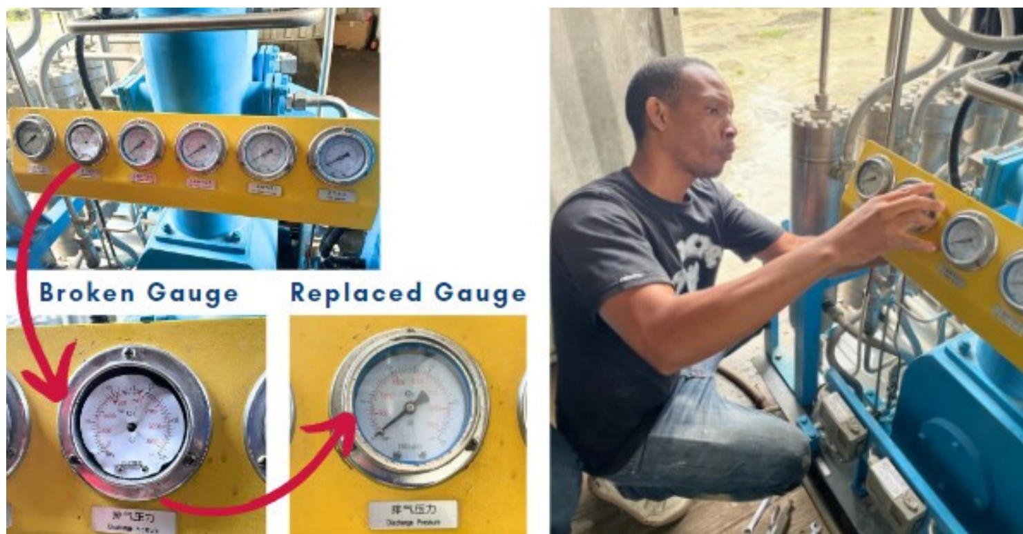
Discharge pressure gauge replacement by biomedical apprentice Weederson in Hinche.
